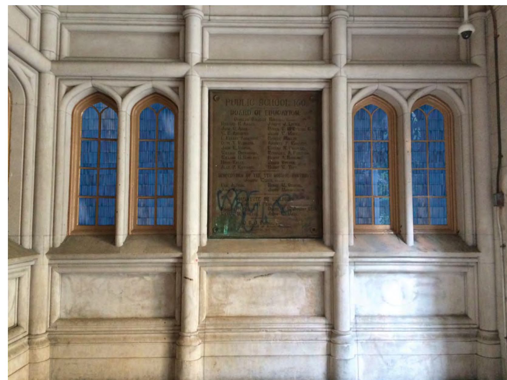
3 View through existing vestibule to new vestibule
