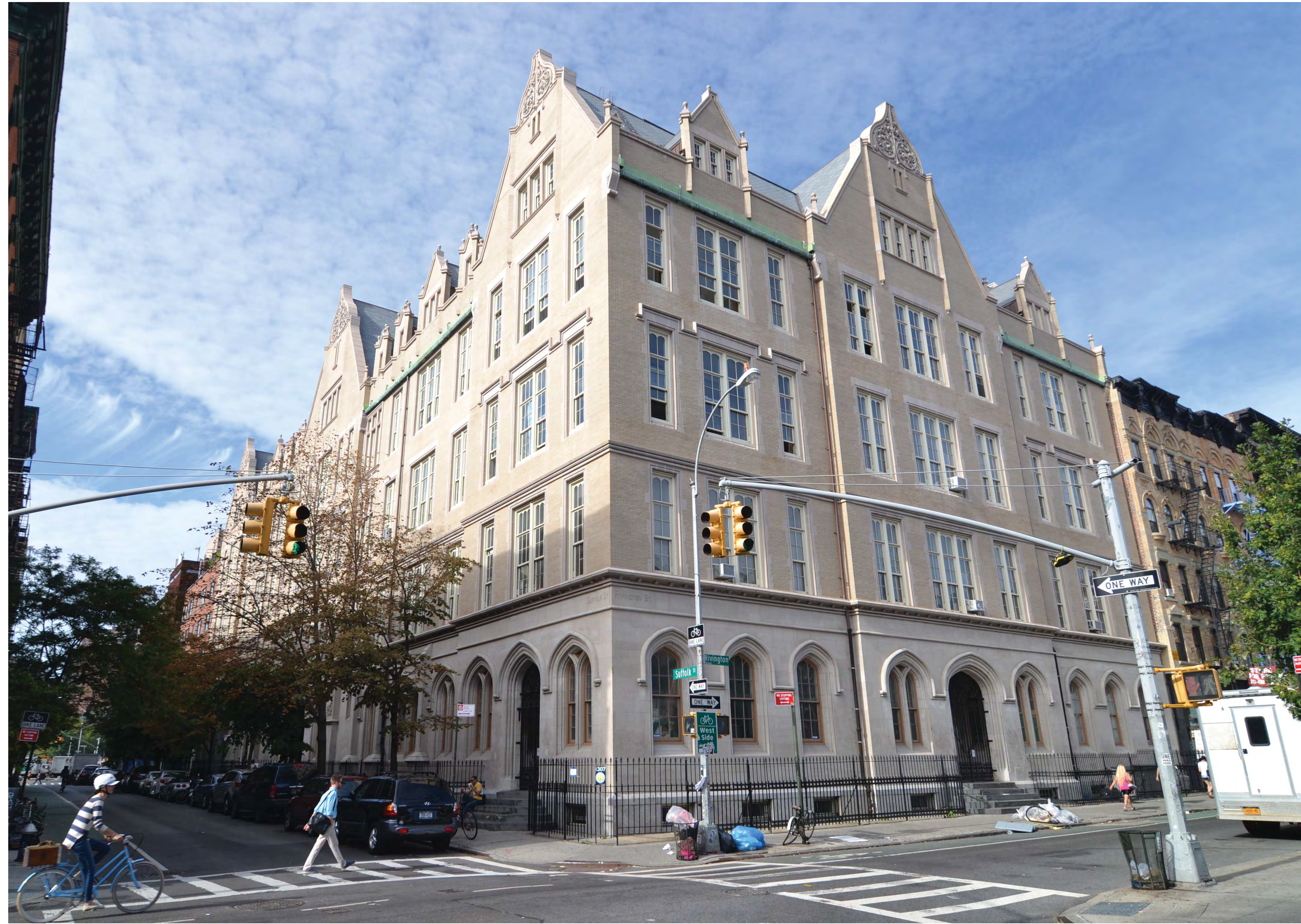
1 Suffolk/Rivington Looking Southwest
