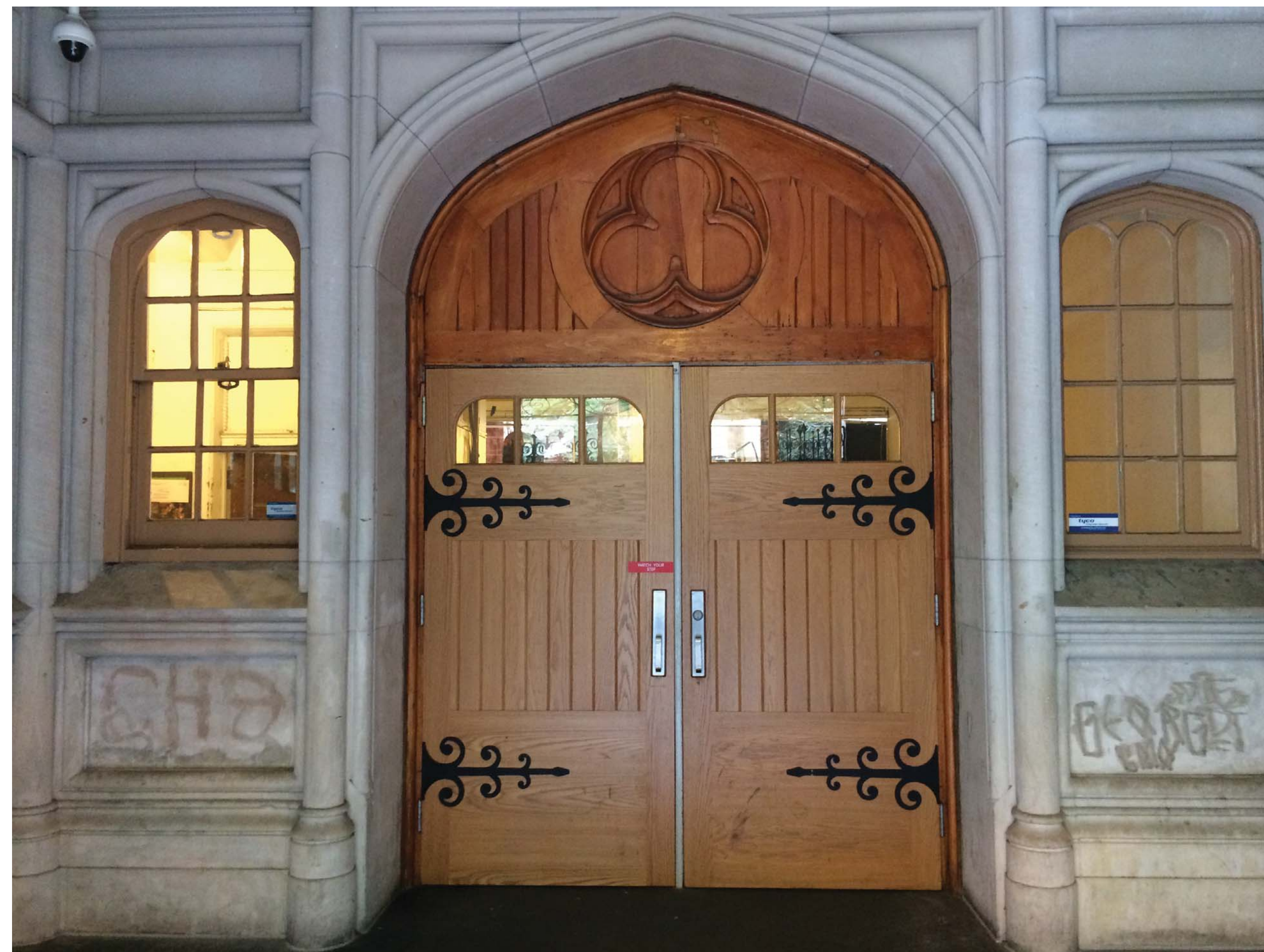
1 Stair Entry West
