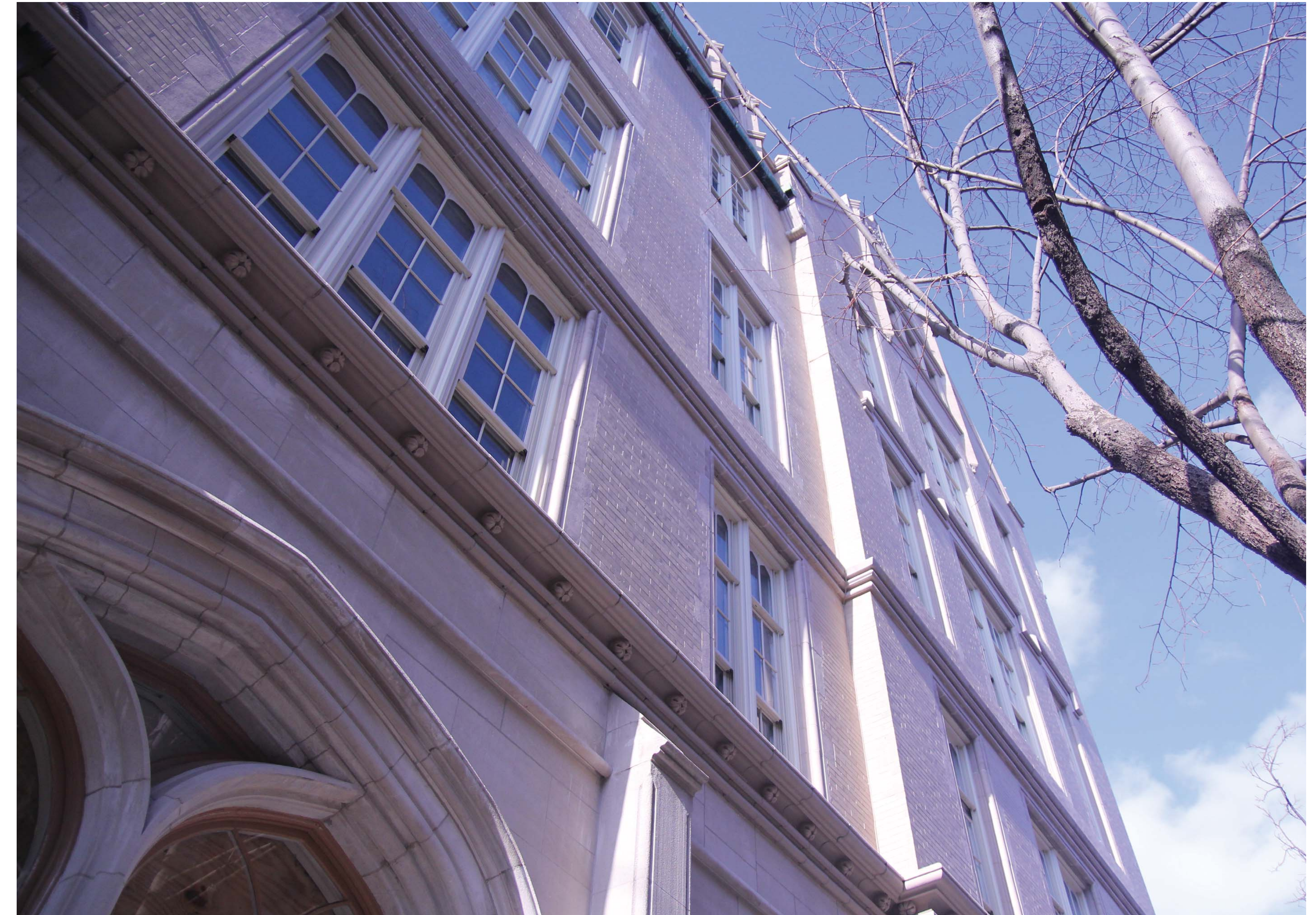
2 Northeast corner, looking up
